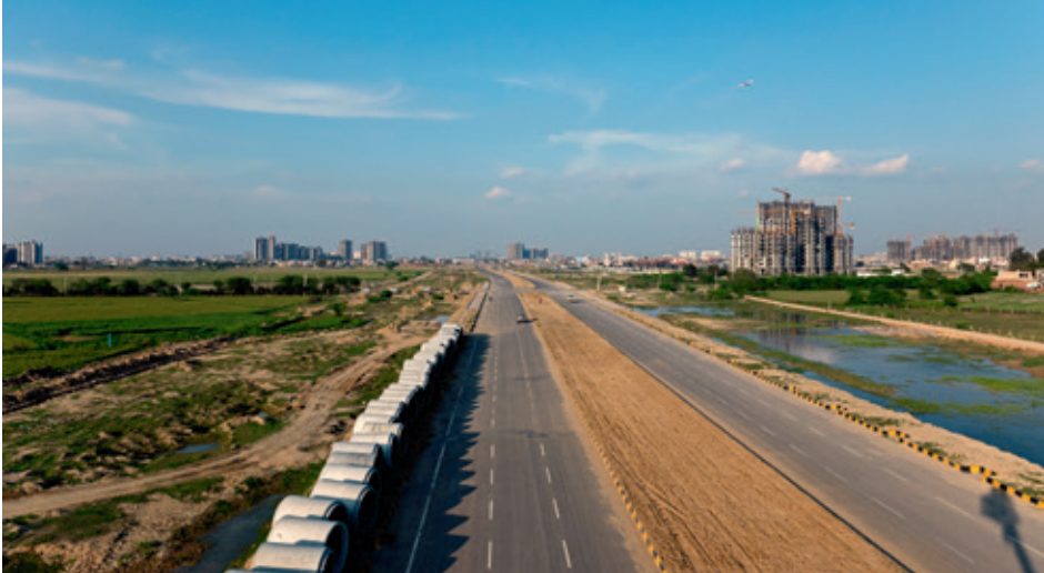
Sewerage pipes being laid along the Expressway
