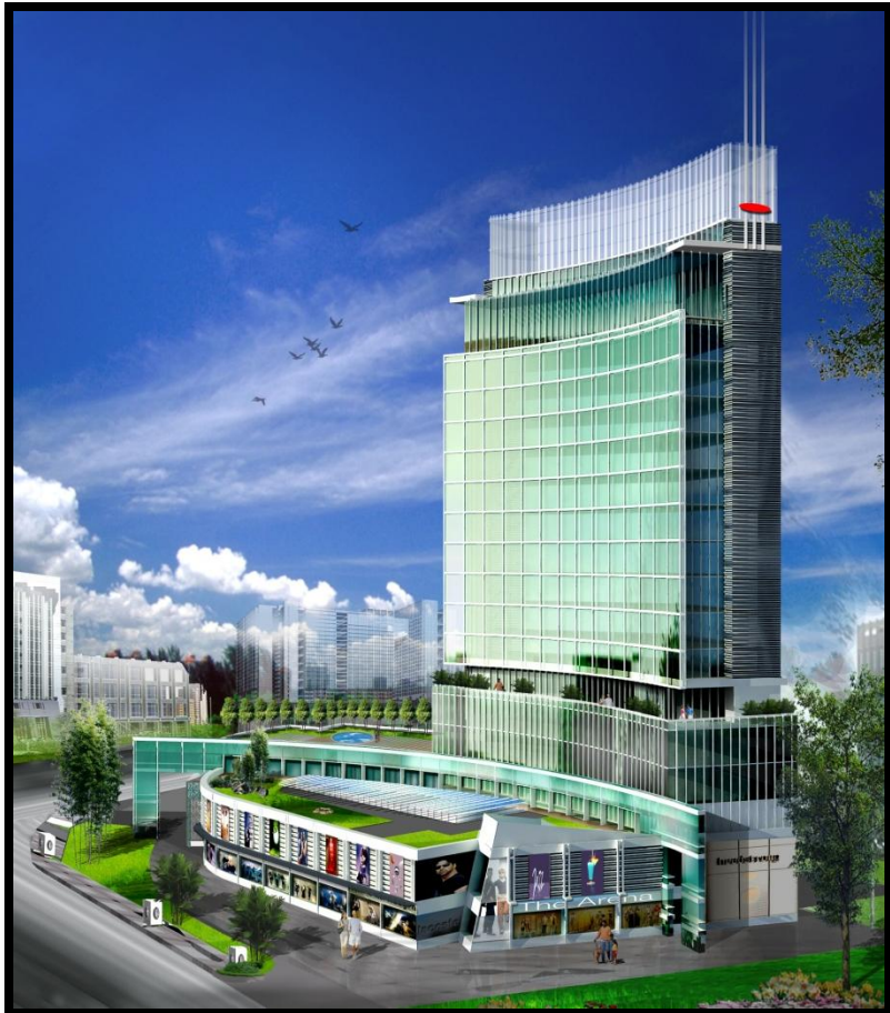
Corporate Tower, Sector-104, Dwarka NPR
